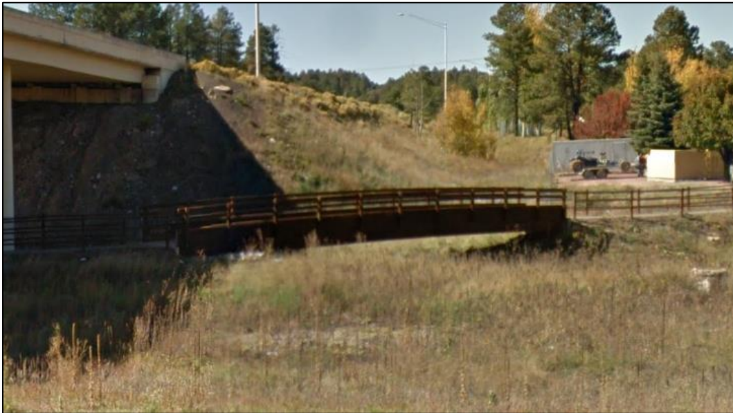
Figure 3: View of Existing Structure from South Beulah Boulevard looking West
